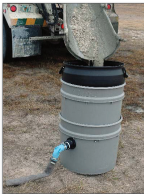
Figure 3. Concrete washout filter
