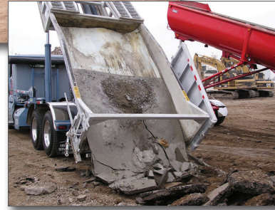
Figure 15. Delivering hardened Concrete to a recycler
