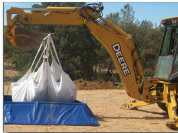
Figure 12. Extracting the concrete solids or gelled washwater
