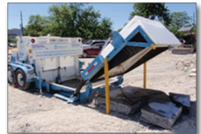
Figure 17. Delivering hardened concrete to a recycler
