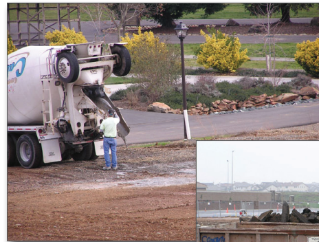
Figure 1. Chute washwater being dumped on the ground
