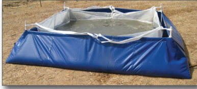
Figure 11. Vinyl washout pit with filter bag
